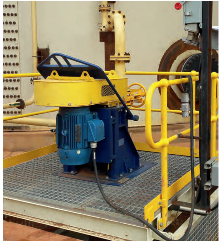
vMAX™ installation with a standard motor mount configuration. Other configurations are available.
